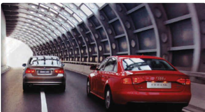
Zhanxi Soundproof Tunnel, China (Skylight) PALSUN® Clear 6mm (3,800sqm)
