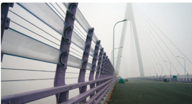
Hangzhou Bay Bridge, China (Thermoformed Wind Shields) PALSUN® 8mm Clear
