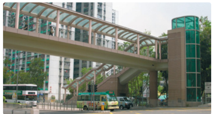
Hung Mui Kuk Footbridge, Hong Kong 6mm Solar-Green PALSUN® Flat Solid Polycarbonate
